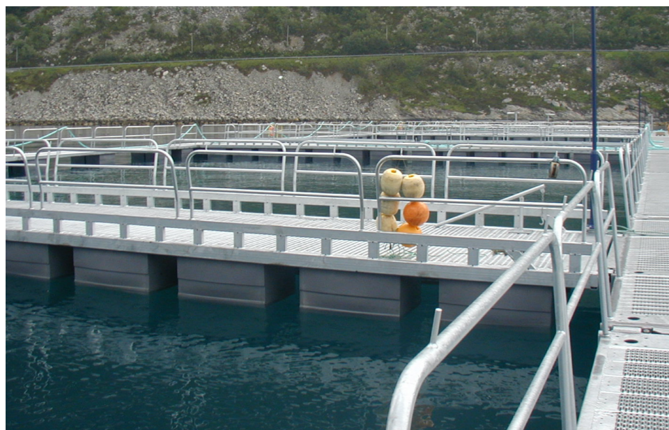
Sections reinforced for forklift driving
